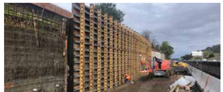
Wall Face Concrete Forming at Retaining Wall No. 2
